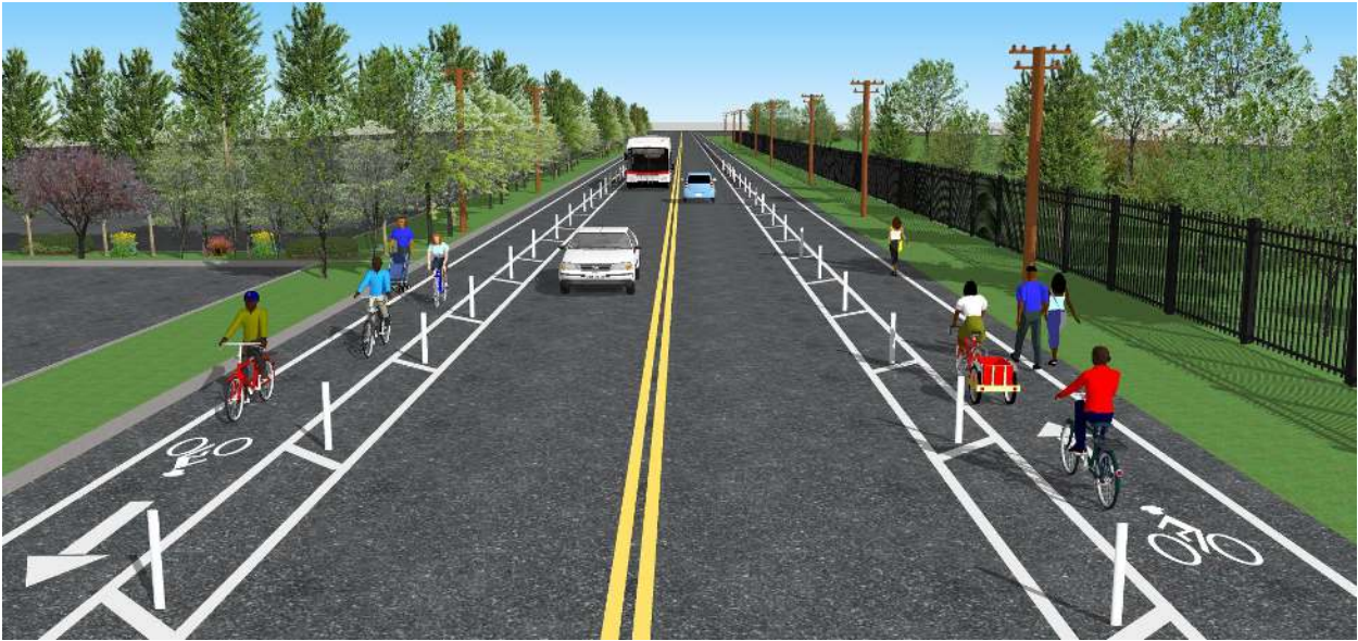
Suitland Road with a Protected Bike Lane
