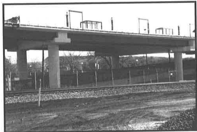
Pedestrians regularly cut across CSX tracks to access the pedestrian tunnel to the Rhode Island Ave Metro station.
