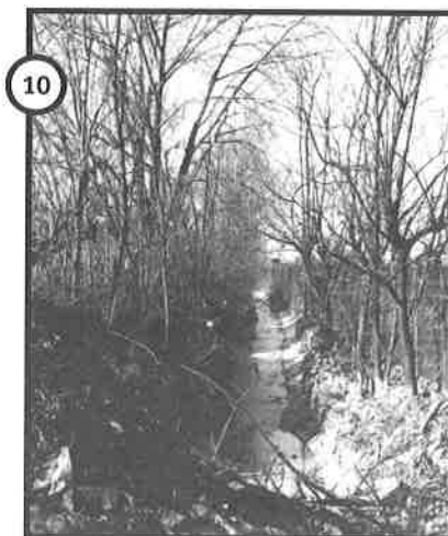
10 A box culvert will be constructed north of Bates Rd. NE, where the trail will parallel Metro through Fort Totten.
