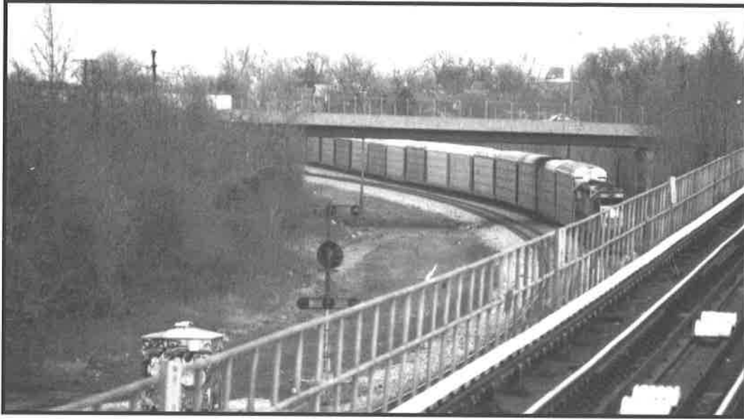
Sections of the trail will parallel an active rail line.
