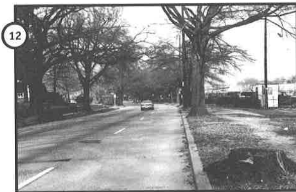
Ultimately, the trail will travel along Blair Rd. for one mile, briefly as a sidepath, then on-road.
